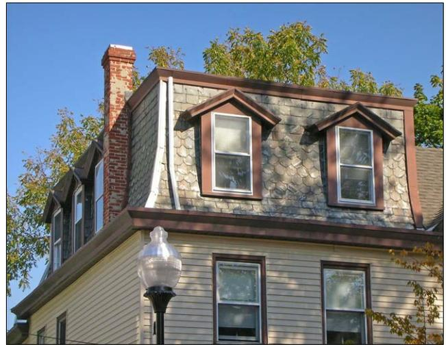
*Mansard roofs are typical of the Second Empire mode of Victorian architecture and are very common in Gloucester City. The steeply pitched concave lower roof slope in this example retains its alternating bands of square and scalloped slates, providing additional texture and visual interest.*
