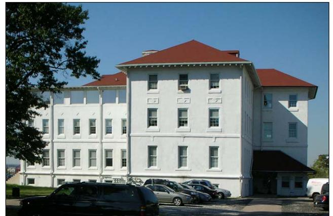
*This building's shallow hipped roof has deep overhanging eaves with projecting rafters that cast strong shadows on the stucco wall below.*
