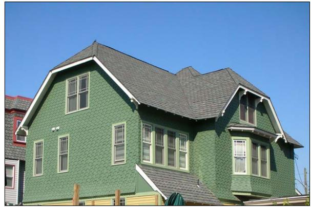
*The cross gables at this roof terminate in jerkin-heads, forming a small hipped roof at the gable end. The deep eaves are supported with decorative wood brackets. Also note that the previous roofing has been replaced with dimensional asphalt shingles with alternating bands of square and scalloped shapes to simulate slate.*
