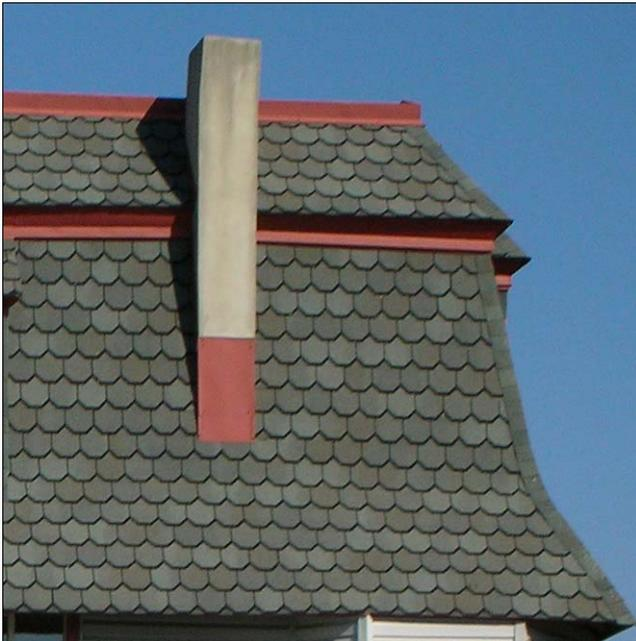
*Dimensional asphalt shingles are available in a variety of shapes and colors to simulate natural roofing materials such as slate.*
