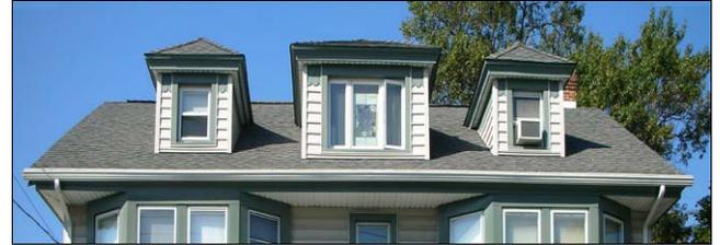
*This side gable roof includes three hipped roof dormers at the front elevation providing natural light and increased habitable space at the upper floor.*
