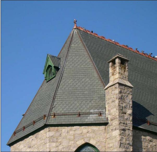
*This roof has a variety of features including the steeply pitched segmented hipped roof with alternating rows of square and scalloped slates; decorative cresting along the top ridge; a copper clad gable roof dormer window; snow guards along the eaves; and a massive stone chimney.*
