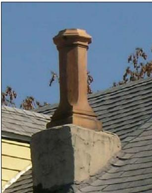
**Chimneys** were typically designed to complement the style of a building and period of construction. In Gloucester City, many are constructed of brick with some stone, some of which have been covered with stucco. Early Georgian, Federal style and Colonial Revival buildings tend towards
