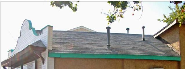
*This commercial building has a decorative parapet at the front elevation that “conceals” a gable roof to the rear. Above the storefront is a pent roof supported by brackets that provides protection from inclement weather for the patrons.*
