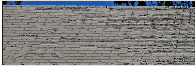
*The surface of the shingles has worn and individual shingles have been dislodged. Roofing replacement should be considered.*
