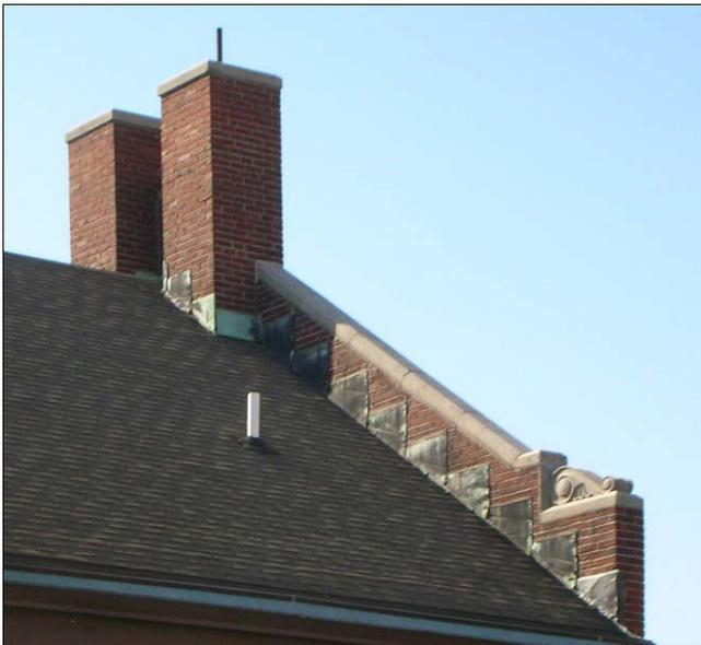
*Stepped copper flashing is visible at the inside face of this parapet wall and the bottom of the chimney. The flashing likely turns under the shingles to prevent storm water from entering in at the edge of the roofing. Also note the pole gutter at the bottom edge of the roof to capture stormwater and direct it towards a downspout.*
